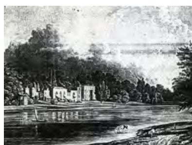
Cross Deep Hall and Riverview Cottage 1828
